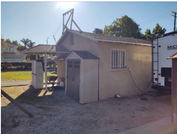
15. Northwest oblique of the garage looking east.
