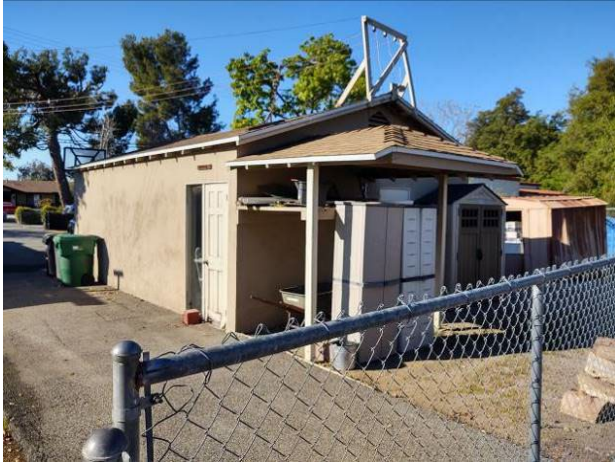
13. Northeast oblique of the garage looking southwest.
