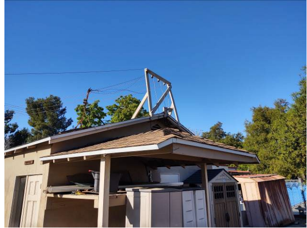
16. Detail of the roof on the garage.
