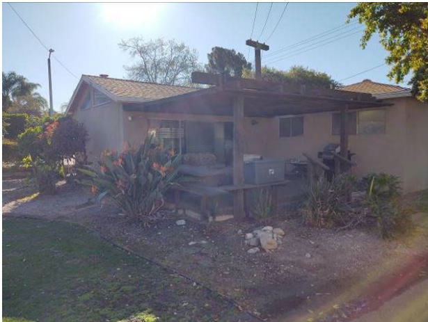
8. Northwest oblique of the rear porch of the main house looking southeast.
