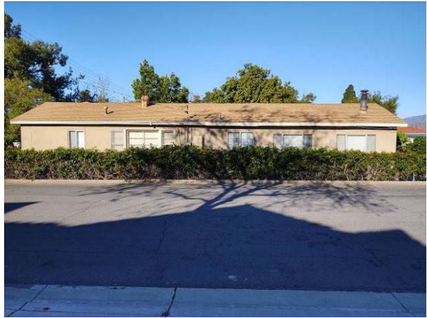
5. East façade of the main house looking west.
