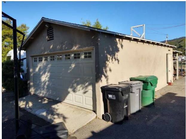
12. Southeast oblique of the garage looking northwest.
