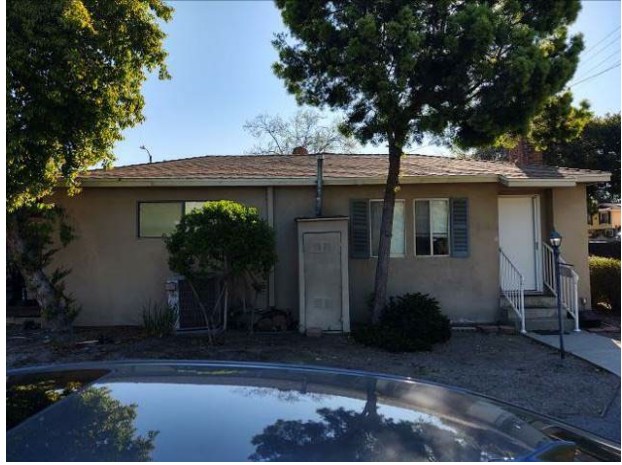
10. West façade of the main house looking east.
