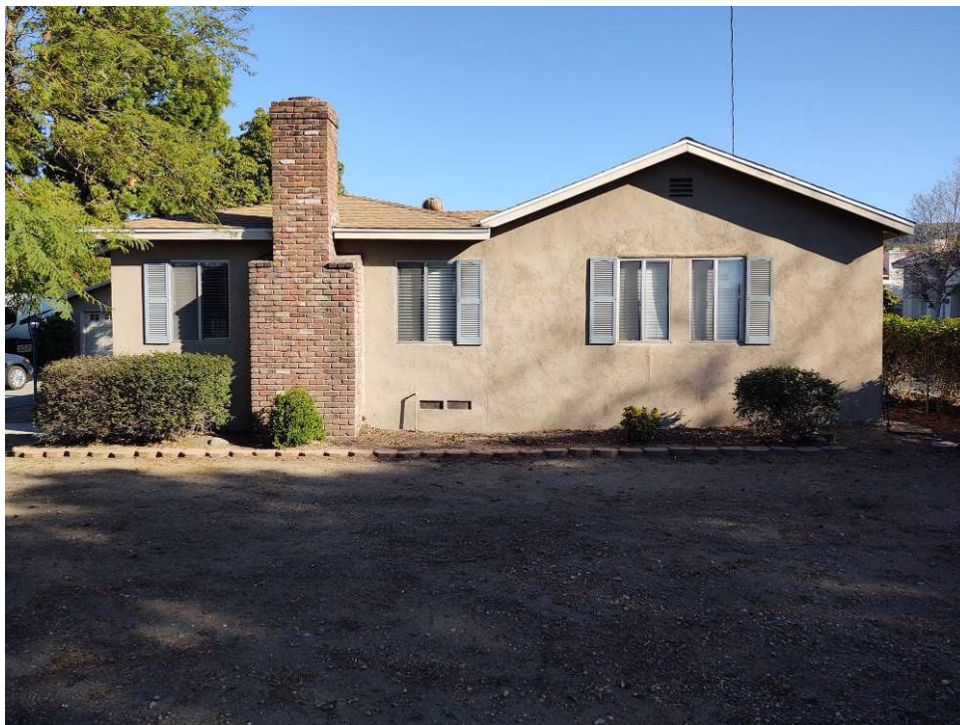
View of the south façade of the main house looking north.
