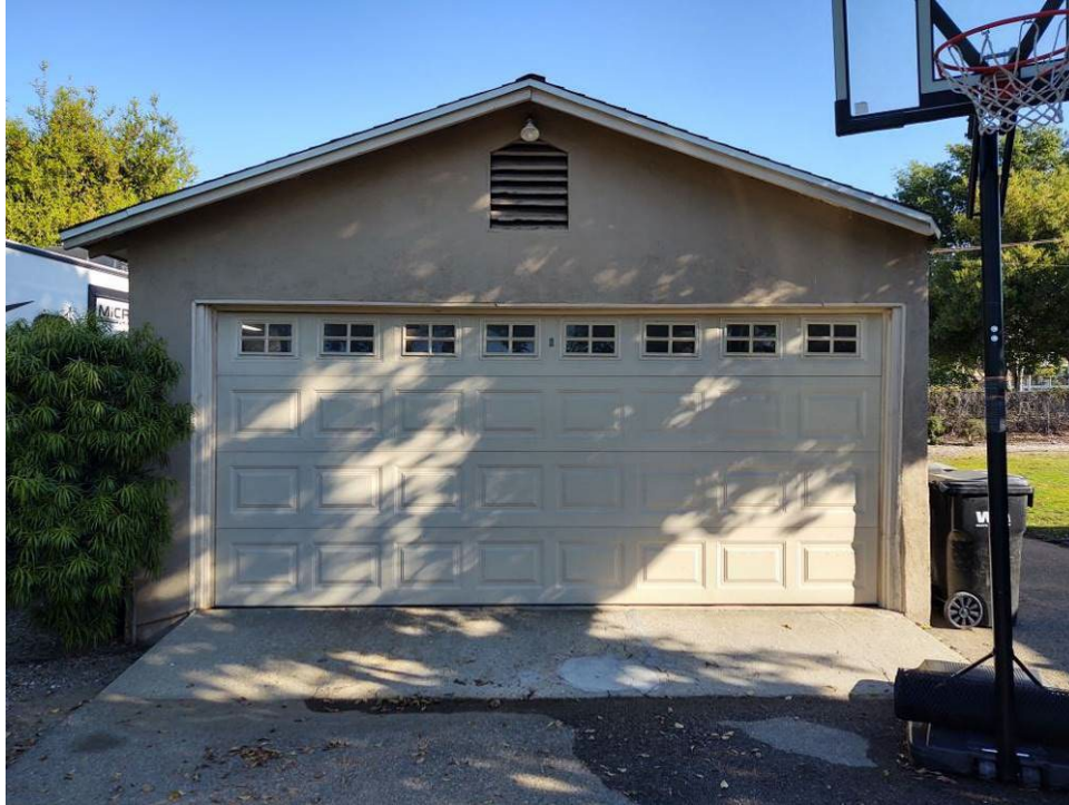
View of the south façade of the garage looking north.
