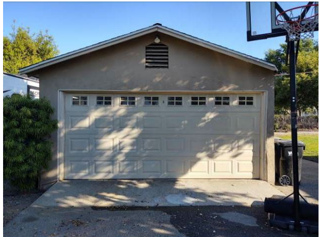
11. South façade of the garage looking north.
