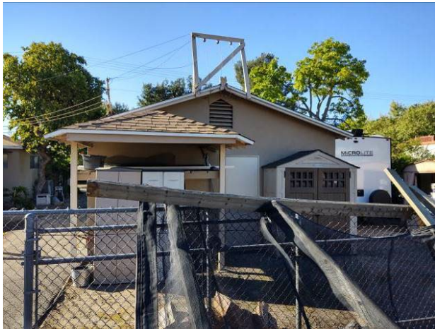
14. North façade of the garage looking south.
