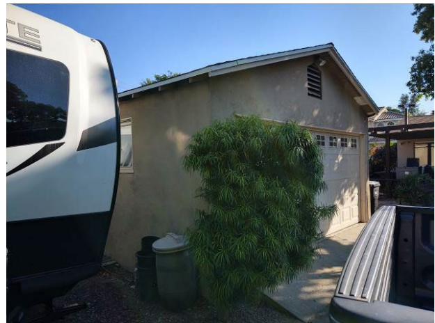
18. Southwest oblique of the garage looking northeast.
