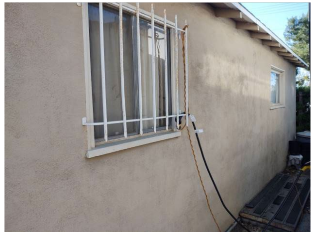
17. West façade of the garage looking southeast.
