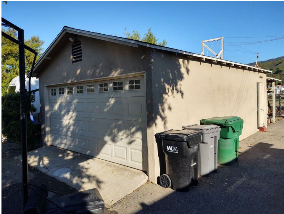
View of the southeast oblique of the garage looking northwest.
