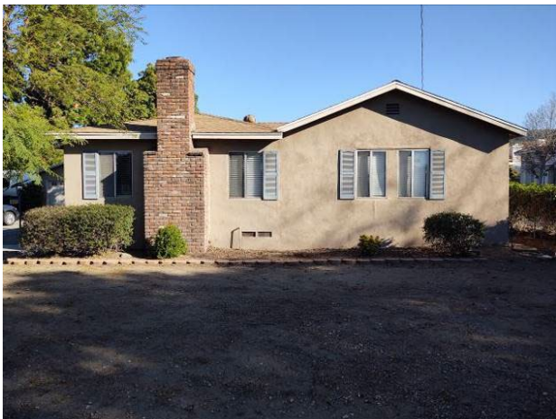
3. South façade of the main house looking north.
